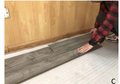
C. Take another long plank, repeat the previous step, insert the long side of plank into long side of previous plank. Then slide plank to your left until the short side is in contact with the short side of the first laid plank.
