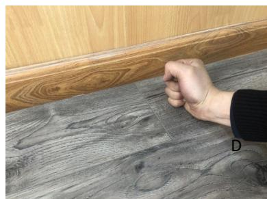
D. Using the drop lock system, drop the short side of the last long plank into the short side of the first laid plank. Slightly tap on the top of the joint of the short side with your fist to secure.
