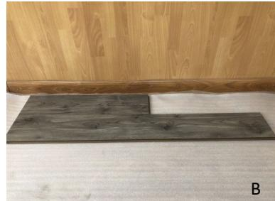
B. The first row must be installed straight. Begin installation back and forth between rows one and two for the first two rows only. Start small plank positioned close to the wall, angle a long plank into the long side of the short plank, and drop long plank tongue into lock. Make sure there are no gaps.
