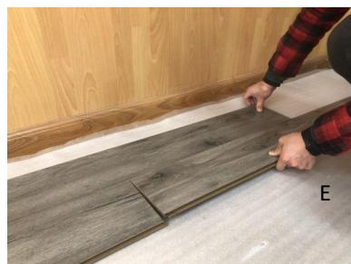
E and F. Finishing rows 1 and 2—continue alternating planks on rows 1 and 2 to avoid misalignment. From row 3 onwards, installation does not require alternating rows. Install one row after the other by starting with angling on the long side, sliding until the short sides are in contact and then locking the short side. As you go, ensure the short sides are securely locked by tap-ping with your fist, or if need be, a rubber mallet.
